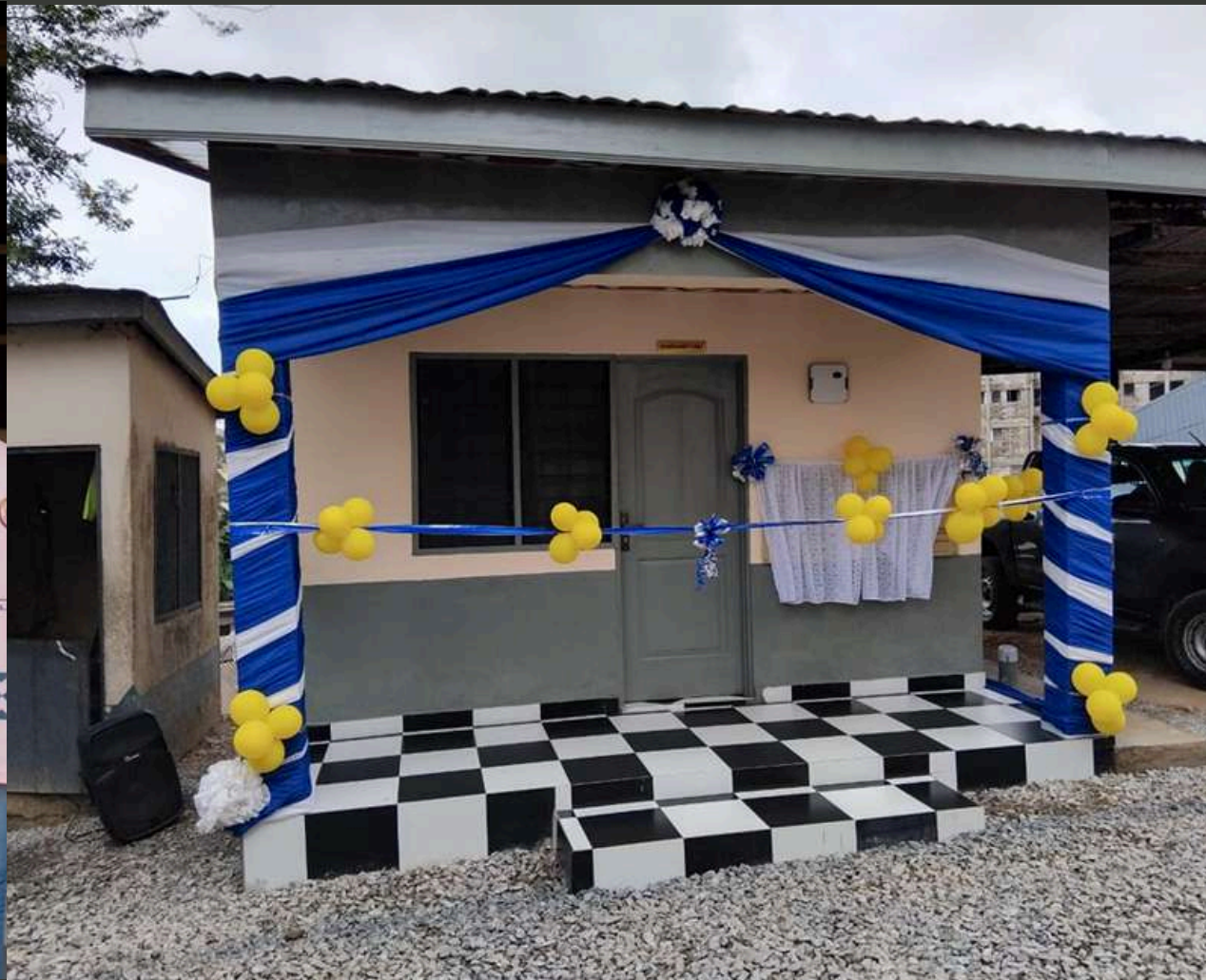
ARDENT FIRE BUILT A CHAPLAINCY OFFICE FOR THE TARKWA LOCAL PRISON
