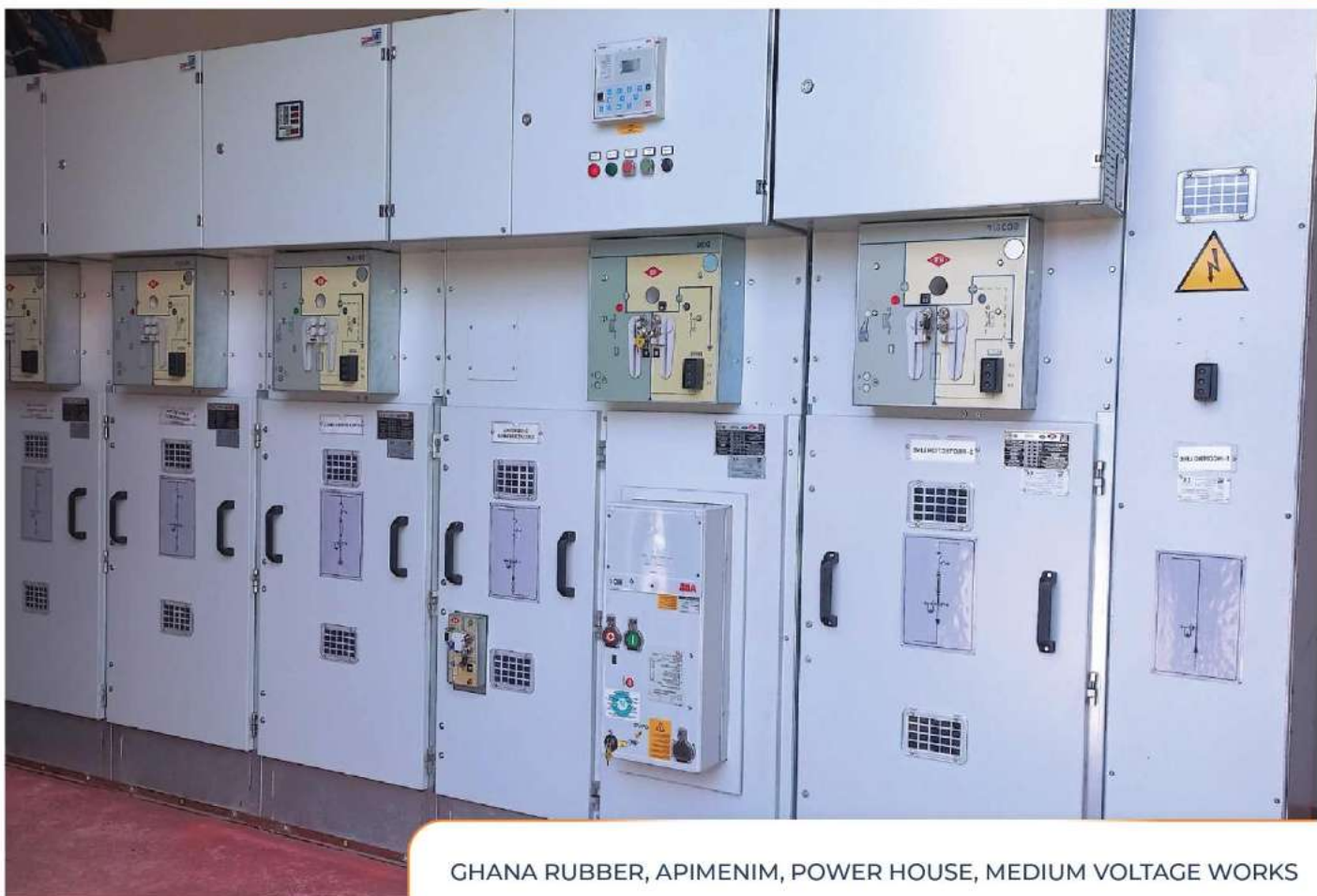
GHANA RUBBER, APIMENIM, MEDIUM VOLTAGE SWITCHGEAR PANEL INSTALLATION
